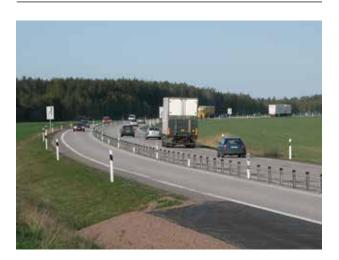
2+1 roads, which alternate two lanes on one side and one on the other every few kilometres, with a dividing barrier between, are part of Sweden's systembased approach to reducing the number of head-on crashes on highways.
