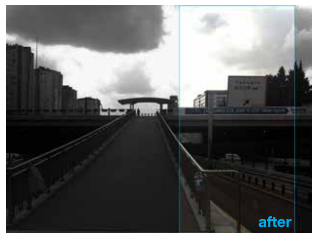
Figure 27 Example of a station where guardrails are placed at the point of interface between over/under-passages and the station platforms to keep people away from the Metrobüs lanes
