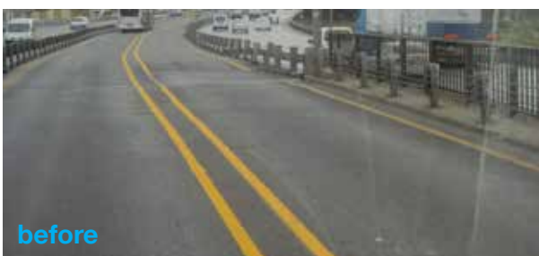
Figure 17 Metrobüs road surface repair-maintenance works
