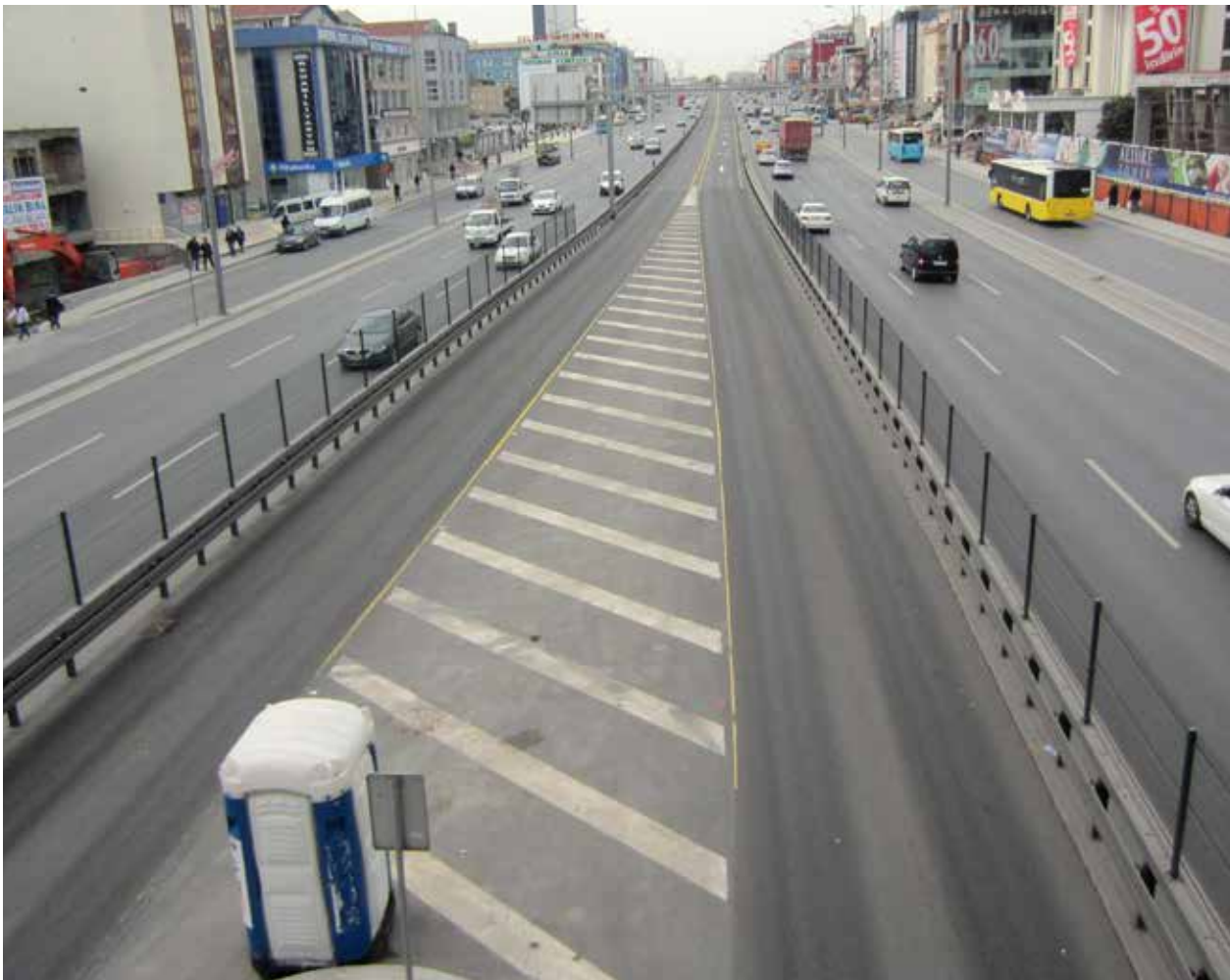
Figure 26 Example of a station where wire fencing stretches to the end of the ghost islands
