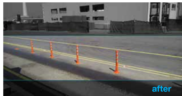
Figure 13 Bollards are placed in some stations so that BRT busses can draw in the passenger platform
