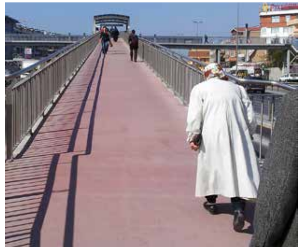
Figure 33 Example of a station where accessibility is improved with ramps for disabled people, elderly people and people with pushchair
