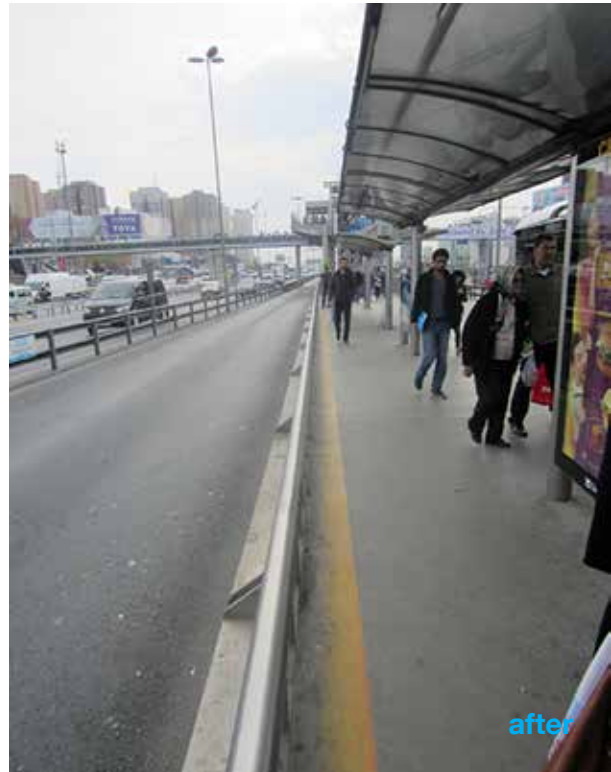
Figure 20 Example of a yellow line marking and surface smoothing
