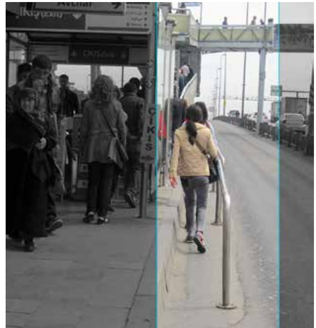
Figure 28 Example of a station where guardrail for passengers is on the road
