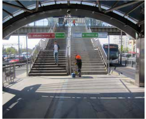
Figure 37 Example of a station where entry and exit gates are separated
