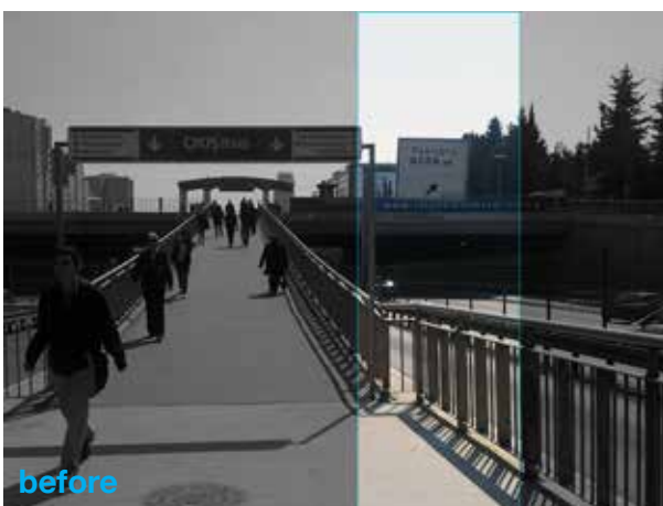
Figure 27 Example of a station where guardrails are placed at the point of interface between over/under-passages and the station platforms to keep people away from the Metrobüs lanes
