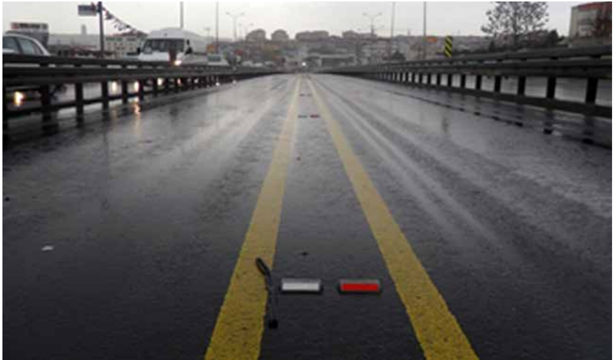
Figure 22 Example of cat’s eyes lay down along the median refuge
