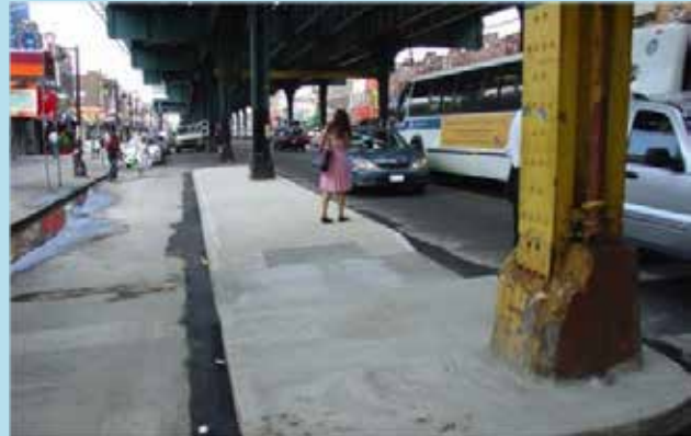
After: 86th Street and Bay Parkway, Brooklyn, NY. Source: New York City Department of Transportation
